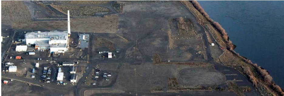
Figure 2: An aerial view of the 324 Building shows its close proximity to the Columbia River.
