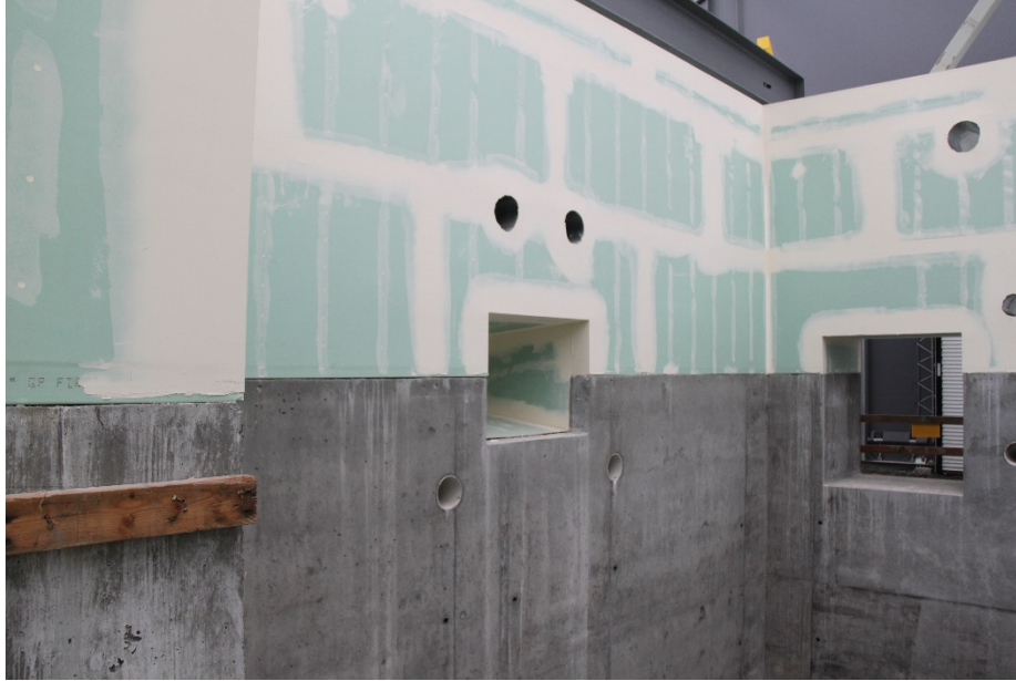
Figure 8: Interior of B Cell mock-up. The square holes in the wall replicate shielded windows; the circular holes above the windows will allow for the eventual installation of manipulators to allow operators remote access into the B Cell.
